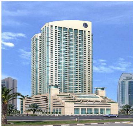
DALMA TOWER ( B+G+40 FLOORS) PLOT A-314.005, TECOM DUBAI MARCH 2005
