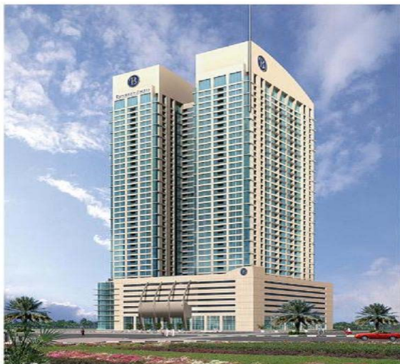
AL YASSAT TOWER ( G+40 FLOORS) PLOT C-201.055, TECOM DUBAI MARCH 2005
